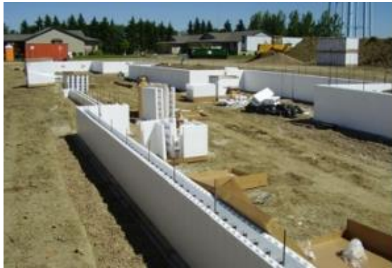
Speed of construction and inherent insulation make ICF cost comparable to other types of below grade applications
